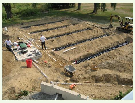
The middle grey water is what leaves the tank and enters a system that can be either lateral lines that are buried into the ground (pictured above), a lagoon system that works like a pond, or countless other system types.
